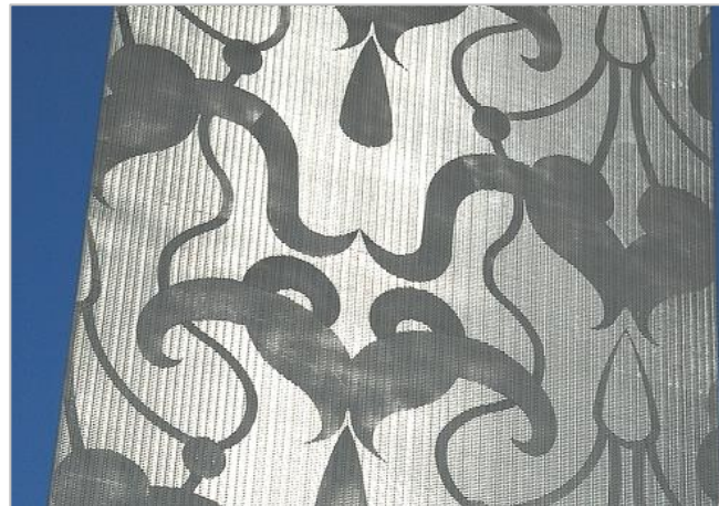
Picture 2: By means of a special etching technique the mesh was decorated with ornaments.
