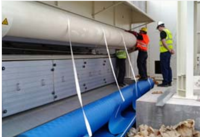
Picture 5: GKD's feeder for the initial installation of belts.
